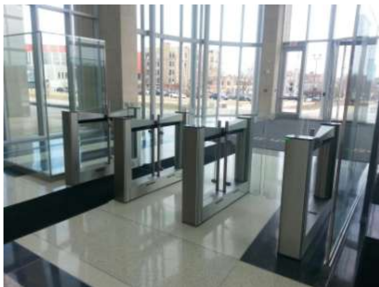
Exhibit 1 Security access turnstiles viewed from side providing egress. (Photo courtesy of U.S. General Services Administration)
