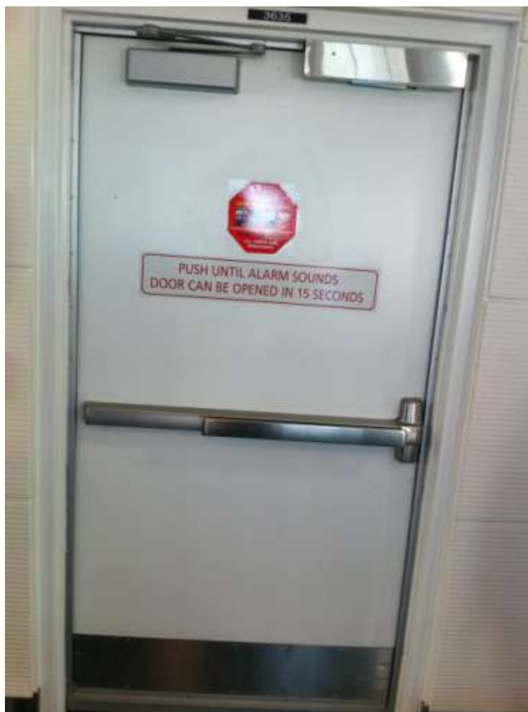
Exhibit 5 Delayed-egress locking hardware.
