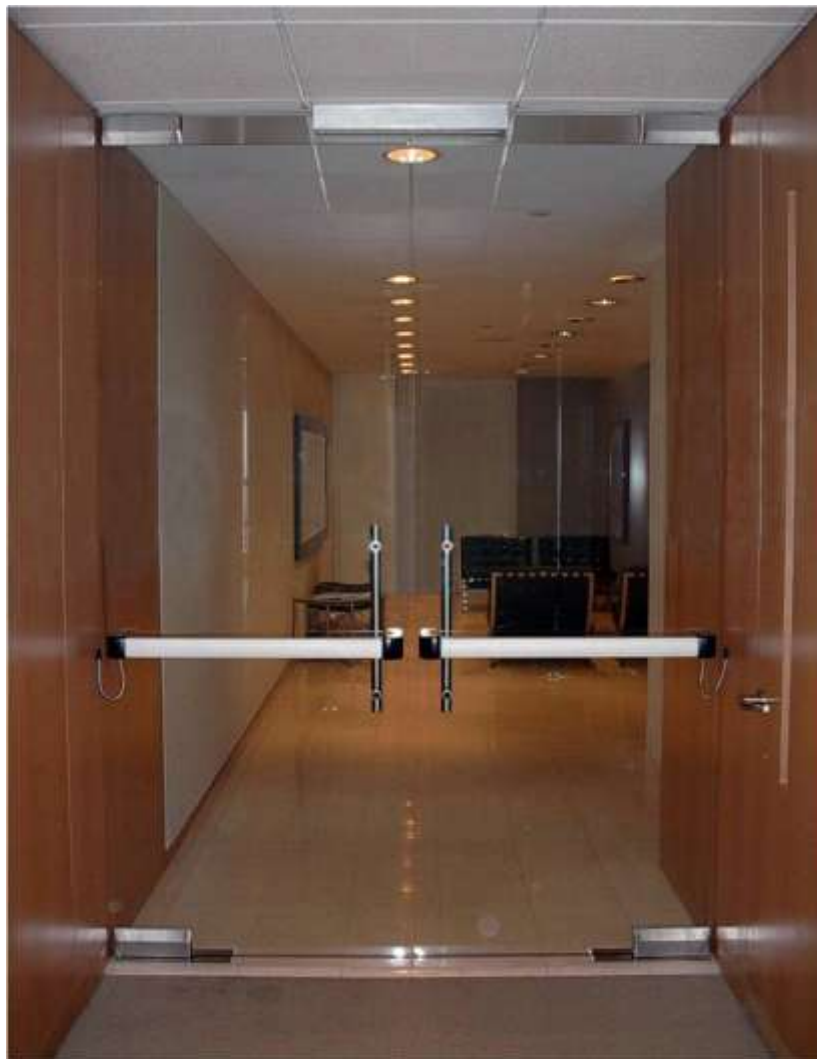
Exhibit 2 An electrically controlled egress door assembly viewed from side providing egress.
