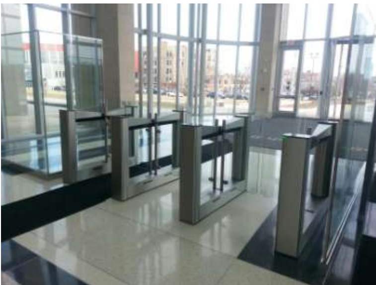
Exhibit 1 Security access turnstiles viewed from side providing egress. (Photo courtesy of U.S. General Services Administration)
