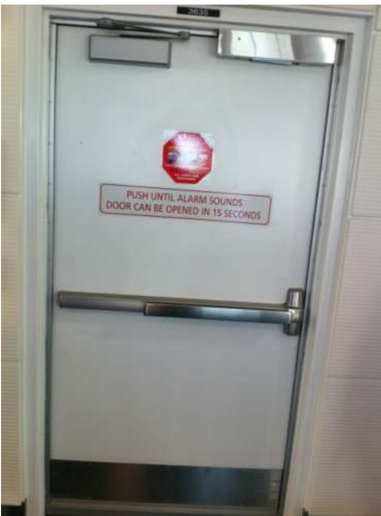
Exhibit 5 Delayed-egress locking hardware.
