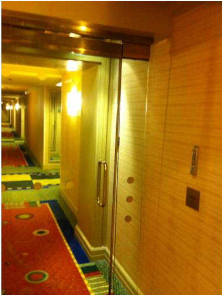
Exhibit 3 Non-egress side of access-controlled door assembly.
