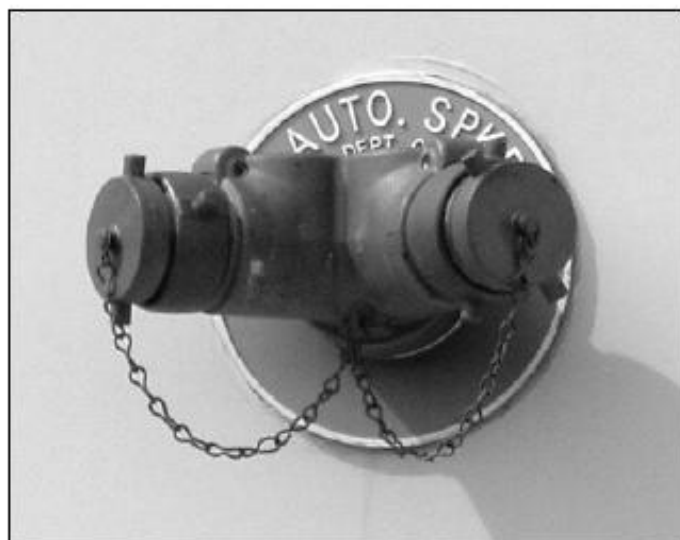
Figure 912.4 FIRE DEPARTMENT CONNECTION WITH SIGN
