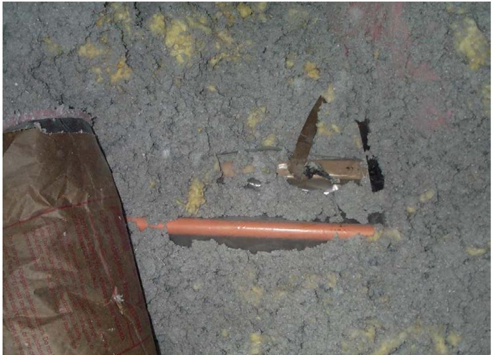
*Tented sprinkler pipe was exposed during maintenance, making it susceptible to freezing in the winter.*
