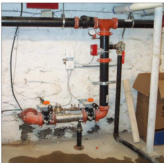
line. Discussions were held in hopes of allowing the use of the domestic line to supply the sprinkler. Unfortunately, since most of the houses were quite old the domestic line was not large enough to support a sprinkler system. The separate water line allows the water authority to shut off the domestic line for non-payment and continue to provide protection for the sprinkler.
