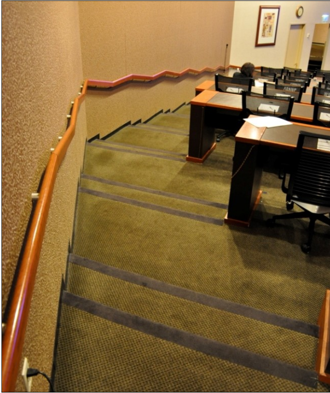
Exhibit 3. Stepped aisle nosing marking accomplished with permanent flooring material. (Photo courtesy of Jake Pauls)
