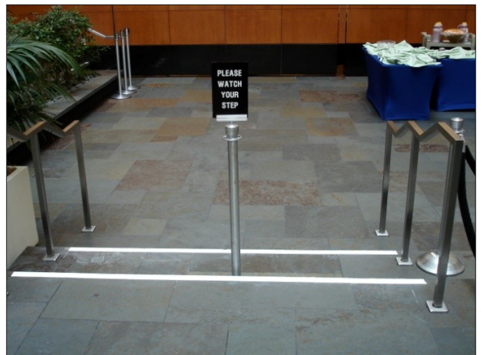
Exhibit 5. Small elevation change effectively marked with striping tape and caution sign. (Photo courtesy of Jake Pauls)
