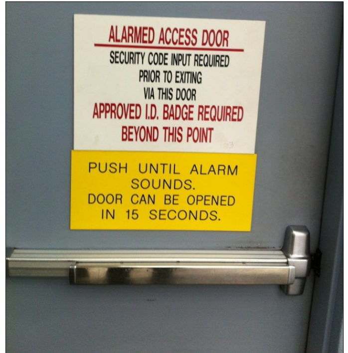
Exhibit 7. Door with delayed egress hardware and conflicting information placards.
