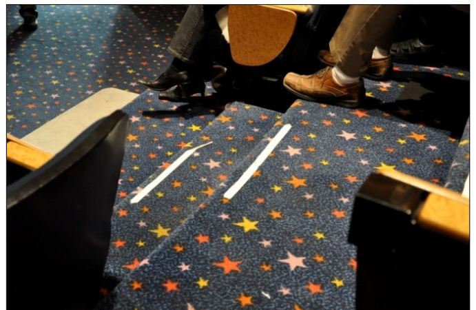
Exhibit 2. Stepped aisle nosing marking attempted with nonpermanent tape. (Photo courtesy of Jake Pauls)
